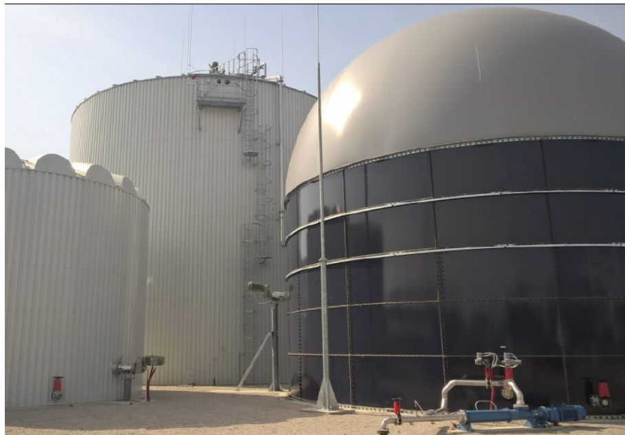
Figure 9: Picture of the biogas plant in Zagreb. From left to right: buffer tank, digester, and post digester/ biogas buffer [6].
